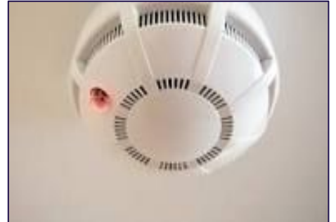
This is a Carbon Monoxide detector..
